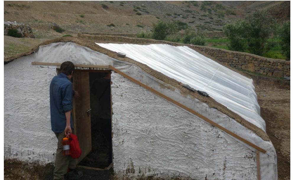
School expedition to the Indian Himalayas: constructing a rammed earth Greenhouse for a remote village
